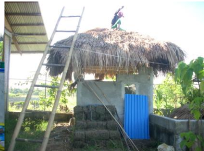
New Dogania pond under construction.
