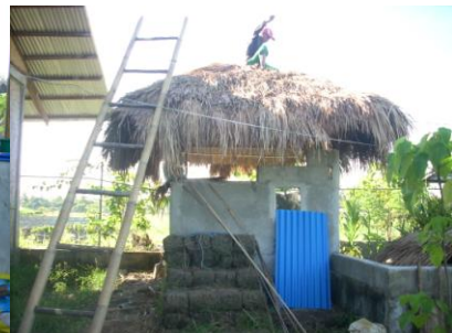
New Dogania pond under construction.
