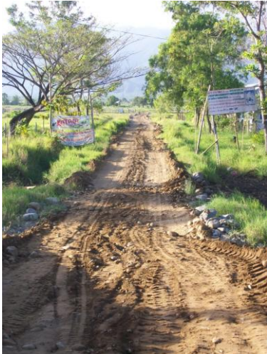
KIEBC access road.
