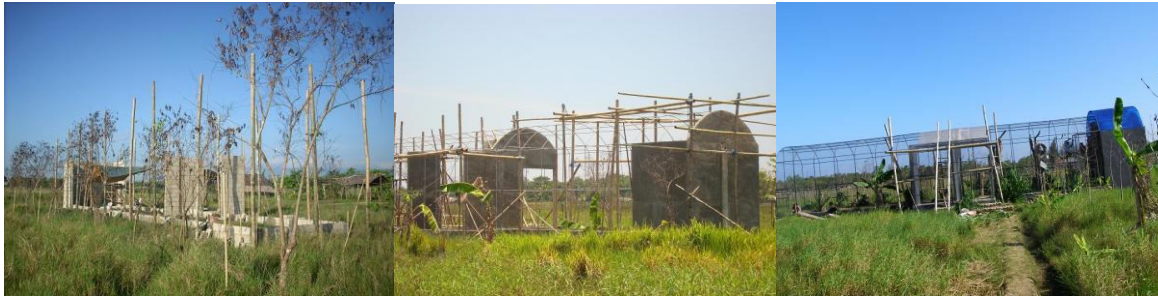
Construction process of the viewing and breeding aviaries for the cockatoos.
