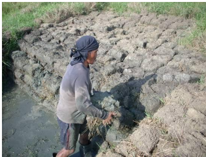
Manual backfilling of mount.
