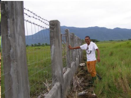
Permanent perimeter fence.
