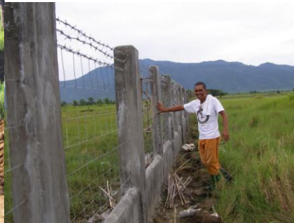
Permanent perimeter fence.
