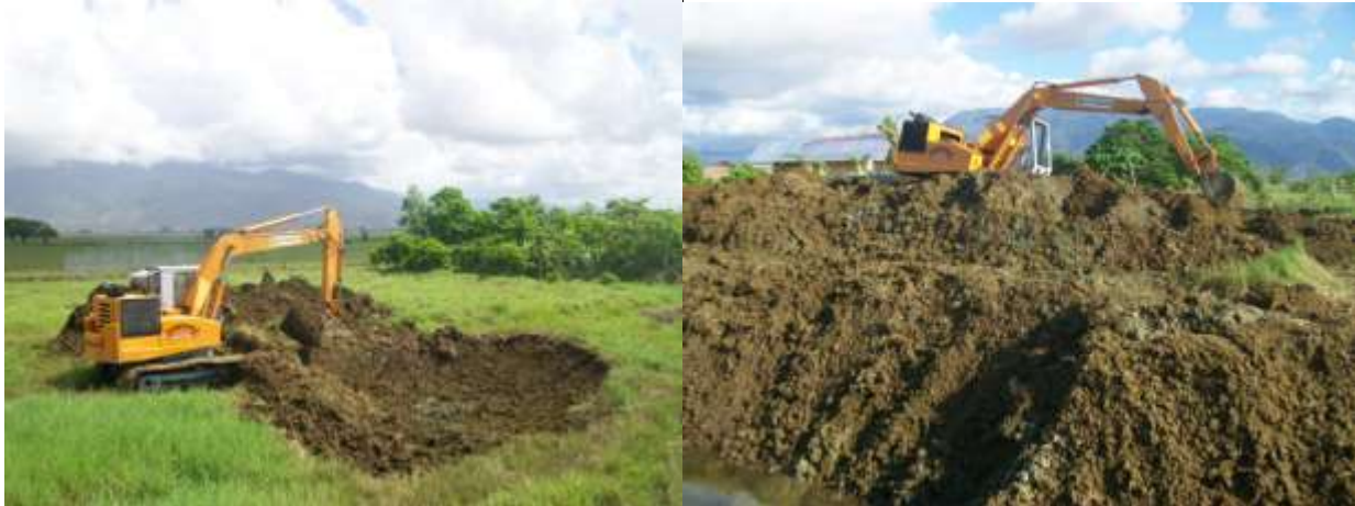
Figure 1: Landscaping with the help of a backhoe in May.
