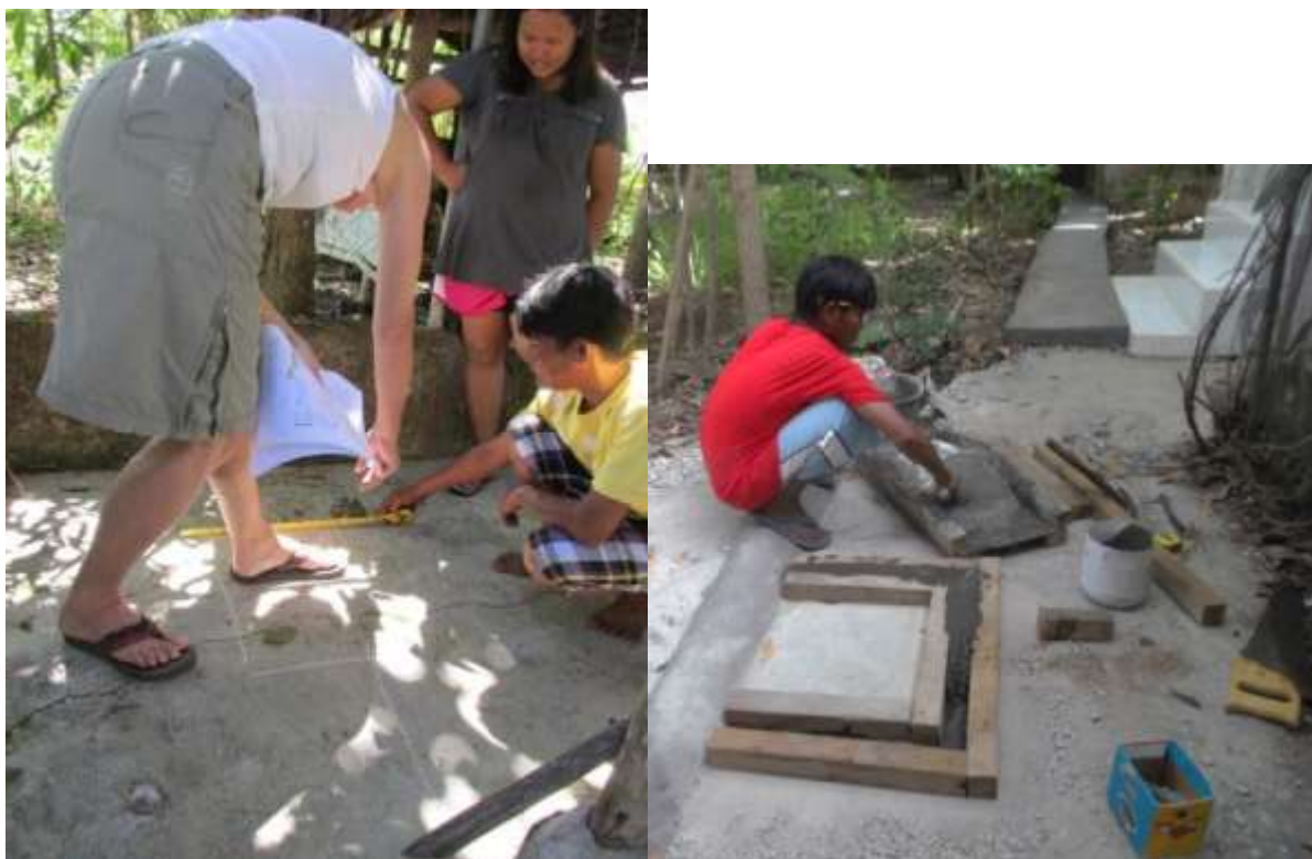
Figure 21: Lay-out of hump and foot bath (left) and pouring of concrete (right).
