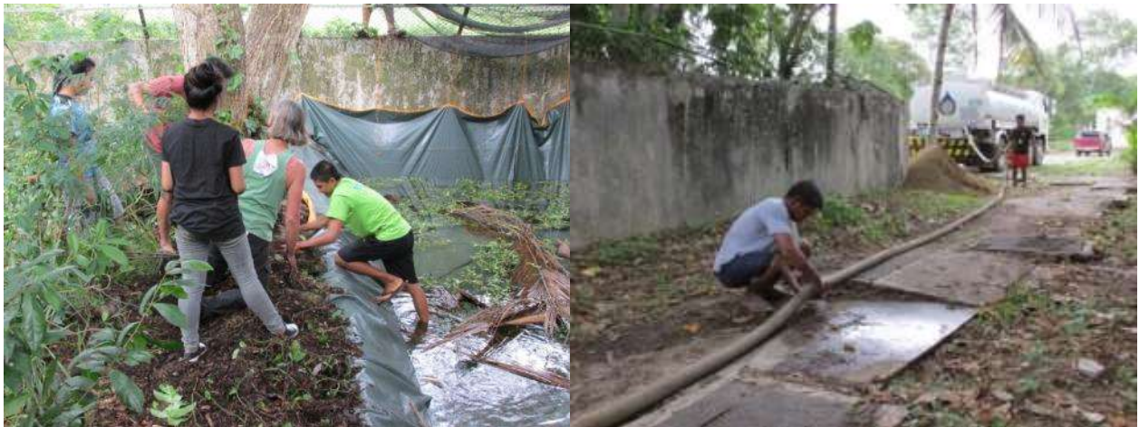
Figure 30: Setting pond liners and nets for shade. Filling with water from the local water district.
