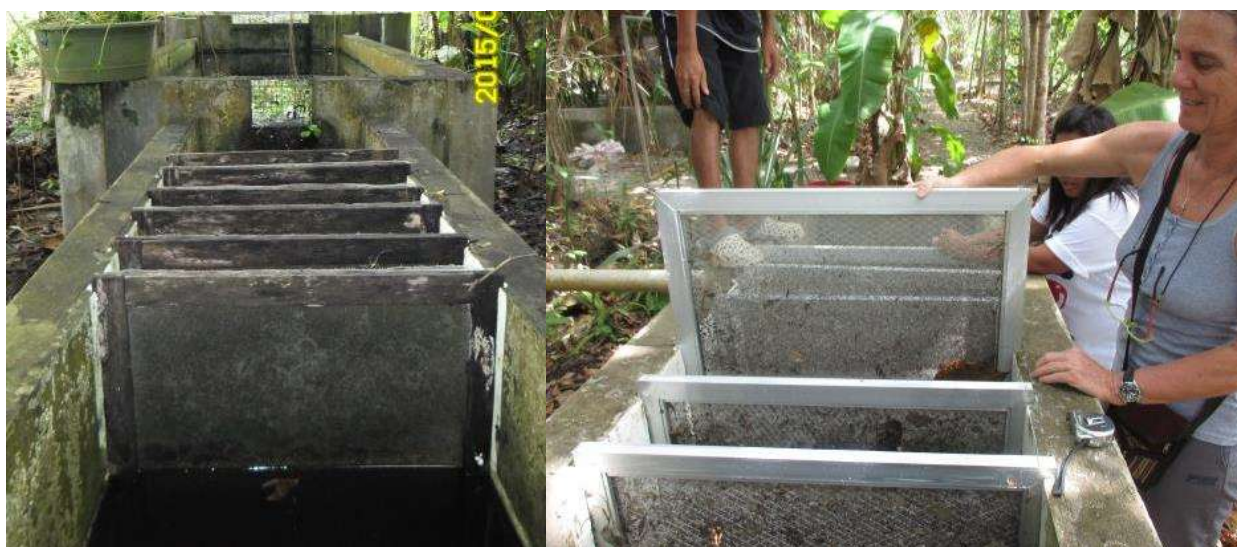
Fig. 24: Old (left) and new filters (right) the water treatment system.
